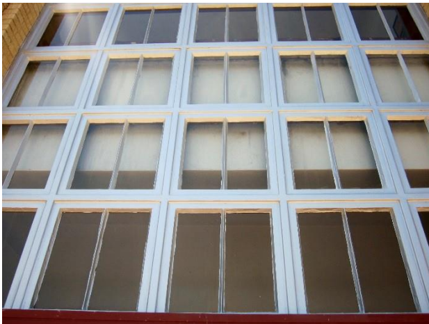
Steel windows above main entry door
