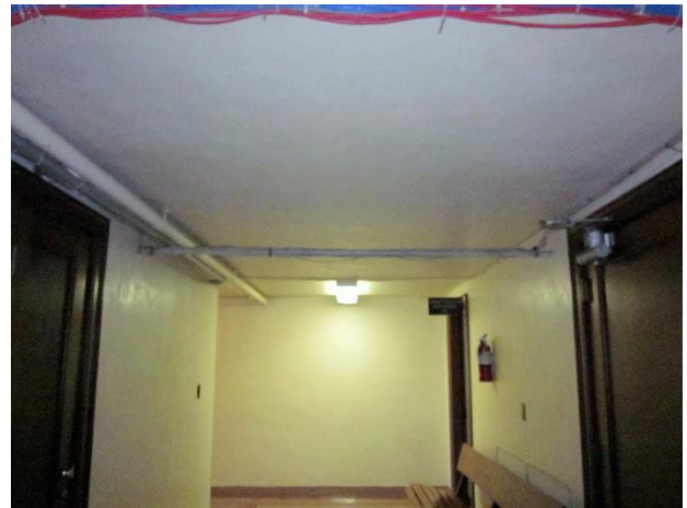
Basement level ceiling
