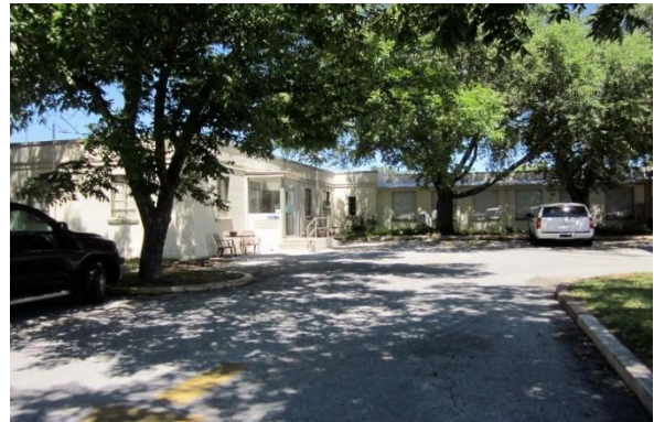
Year Built: 1979 Square Feet: 19,123
