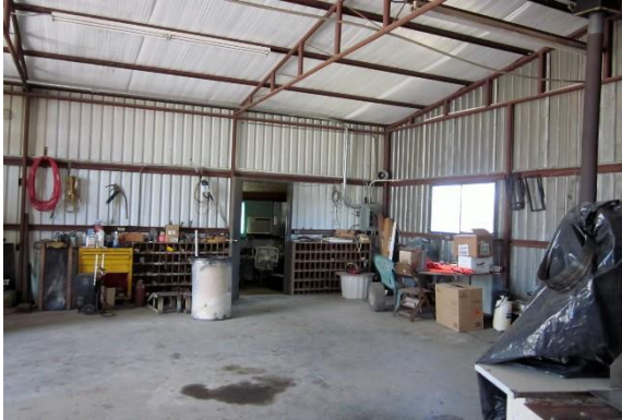
Pct. 2 Barn Interior
