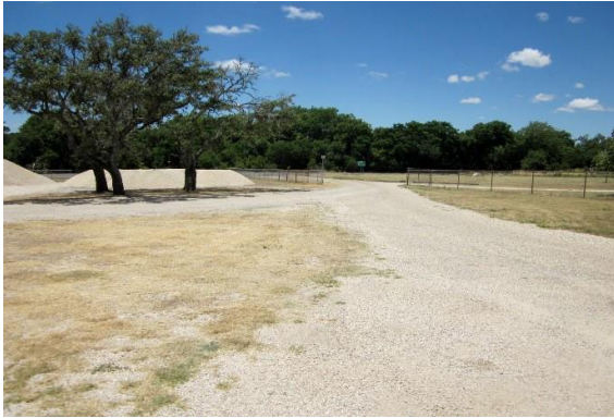
Driveway to County Yard Pct. 2
