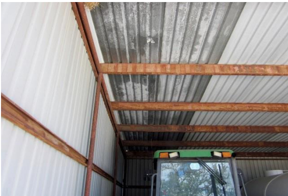
Pct. 2 Barn Interior
