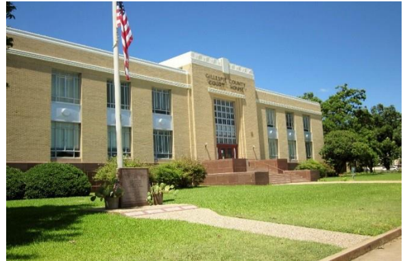
Year Built: 1939 Square Feet: 30,520
