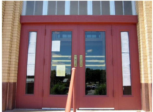
Main entry door
