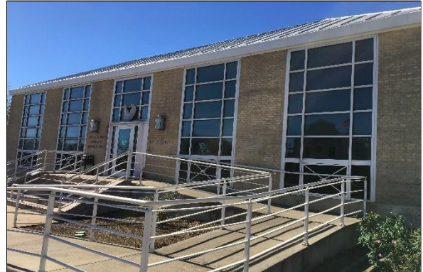
Year Built: 1941 Square Feet: 4,424
