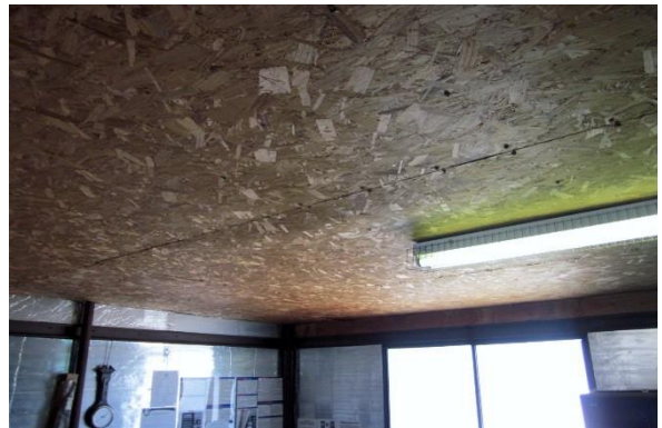
Pct. 2 Office Space Ceiling
